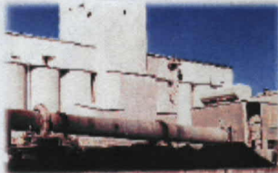
Rotary kiln pictured in foreground
